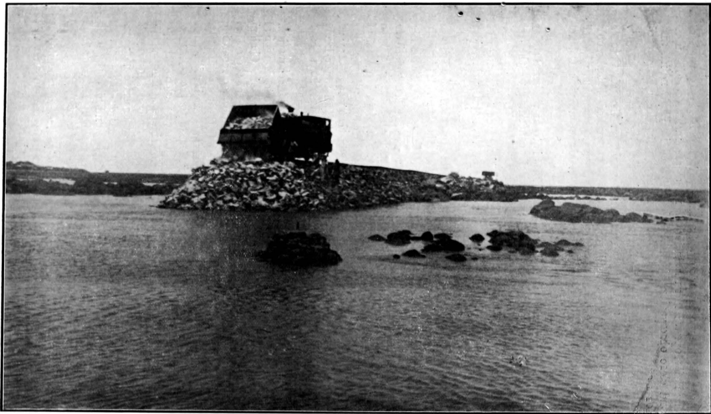
End Tipping Rubble Mound at R. D. 5,500 (From outside).
